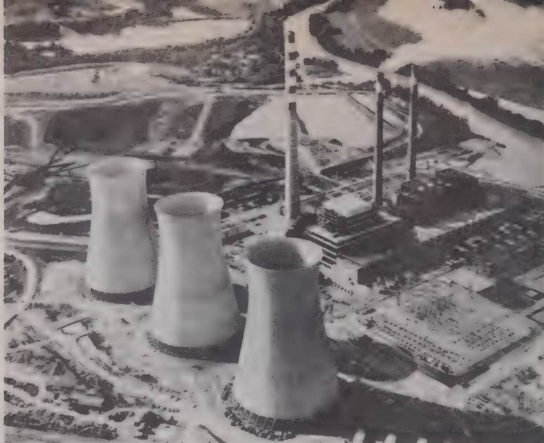
Giant cooling towers were installed at the Paradise steam-powered generating plant in southern Kentucky after the Tennessee Valley Authority found that warm water discharged from the plant into the Green River Reservoir forced fish away from the area.
